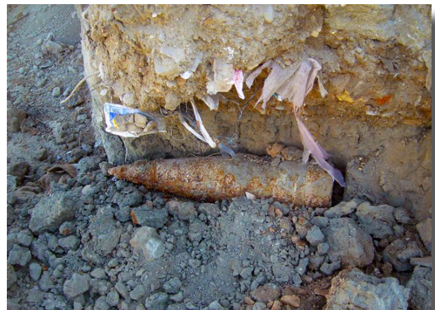
Unexploded ordnance is a common find on a construction site in Afghanistan after years of war. (Official USACE courtesy photo/released. Photo Credit: Todd Lyman)
